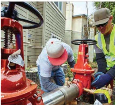
LF009 Reduced Pressure Zone Assembly
