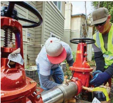
LF009 Reduced Pressure Zone Assembly
