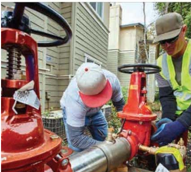
LF009 Reduced Pressure Zone Assembly
